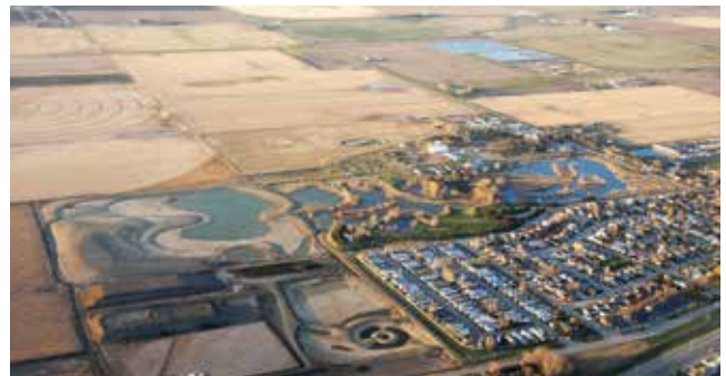
CONSTRUCTED WETLAND—TOWN OF COALDALE
